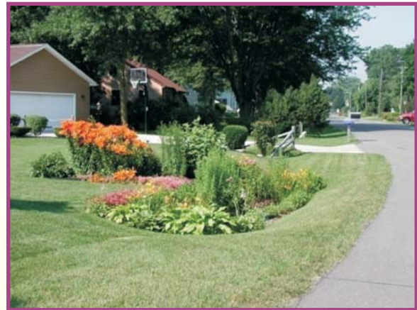
A soil storage and rainwater seepage system
