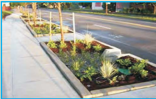
Green Infrastructure to absorb Rainwater that comes from road after rain (Source www.rainwatercollecting.com )
