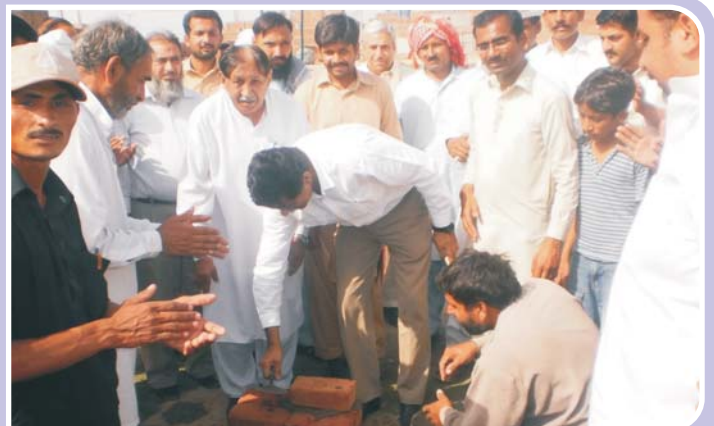
MD WASA Faisalabad laying the foundation stone of water works
